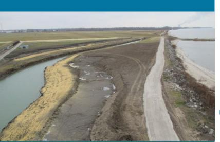
This design-build civil and environmental restoration project required Kwest Group to navigate live firing schedules and unexploded ordinances while repairing and rehabilitating century-old storm drainage and lagoon systems at Camp Perry, Ohio.
