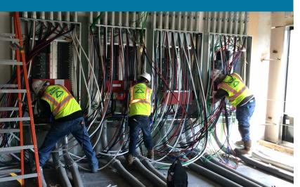
Trio self-performed 90 percent of the electrical work on this six-story office building and five-story precast garage tied into existing structures, also featuring a renovated lobby, 1,750-kilowatt diesel generator and 2000A data center with a modular busway.
